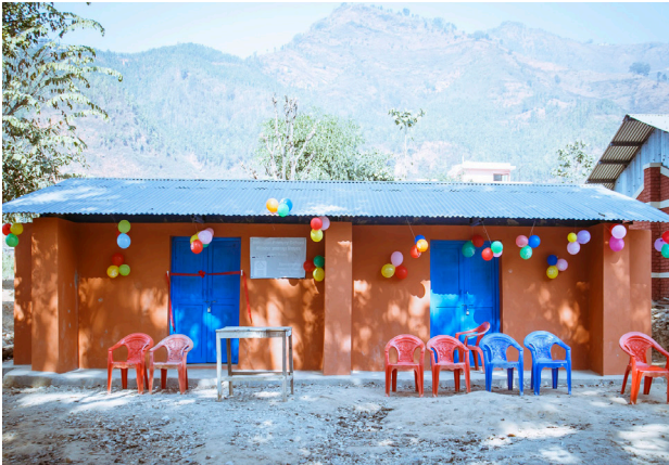
Belingtar Earthbag Primary School, Dhading
